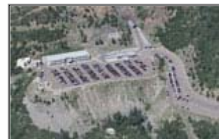
Cheyenne Mountain Air Force Station doesn't look like much from above. That's because the combat operations center — the installation's nerve center — is hidden beneath more than 2,000 feet of granite. Official Air Force Photo by Tech. Sgt. John E. Lasky
